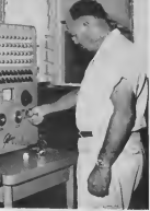
CRUDE FIELD operator Ronald Clauzel flips the calibration switch on the Gilbarco main receiver to check crude level in one of 27 crude tanks so far incorporated in the automatic gauging system. OPERATOR DEN Crude Field Ronald Clauzel in flip a calibration switch arbi e Gilbarco sa receptor mayor pa check nivel di e crudo den e di 27 tankinan cu ya ta inclui den e sistema automatico di gauging.
